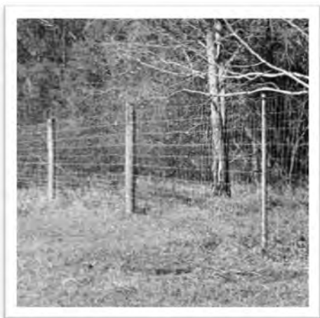
40mm steel post in fence-line
