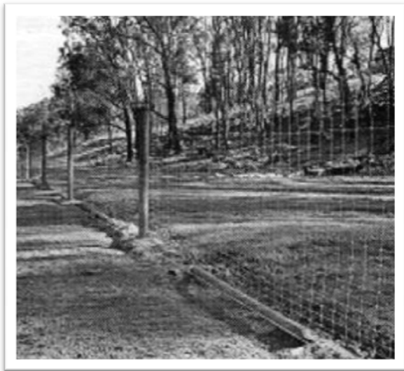
Treated pine posts attached to fence
