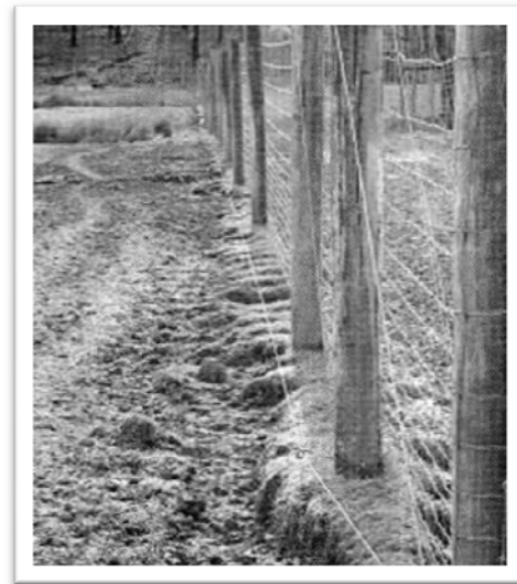
Hot wire at base of fence
