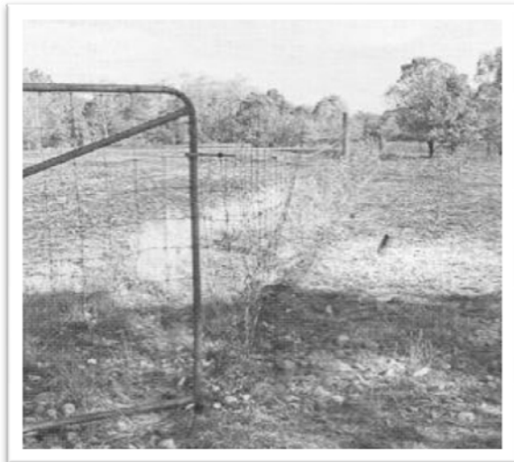
Strainer assembly gone missing. The fence is holding up the gate
